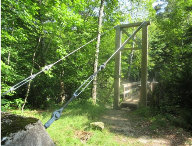
Suspension Bridge on the AT
