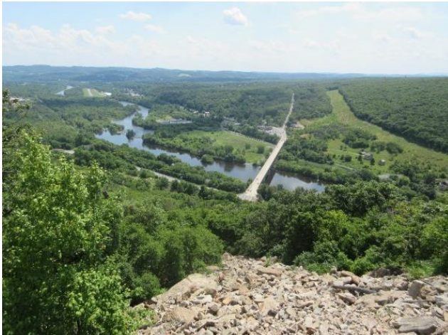
Climbing out of Lehigh Valley (The AT crosses the bridge.)
